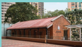
香港大學訪客中心(西區抽水站及濾水廠工人宿舍) HKU Visitor Centre (Workmen's Quarters, Elliot Pumping Station and Filters)
