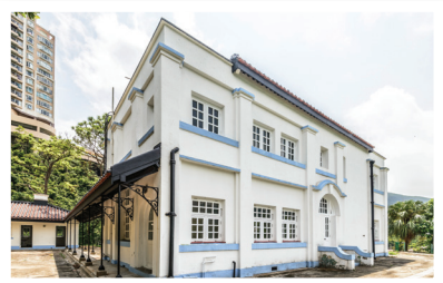
大潭篤原水抽水站員工宿舍群 Tai Tam Tuk Raw Water Pumping Station Staff Quarters Compound
