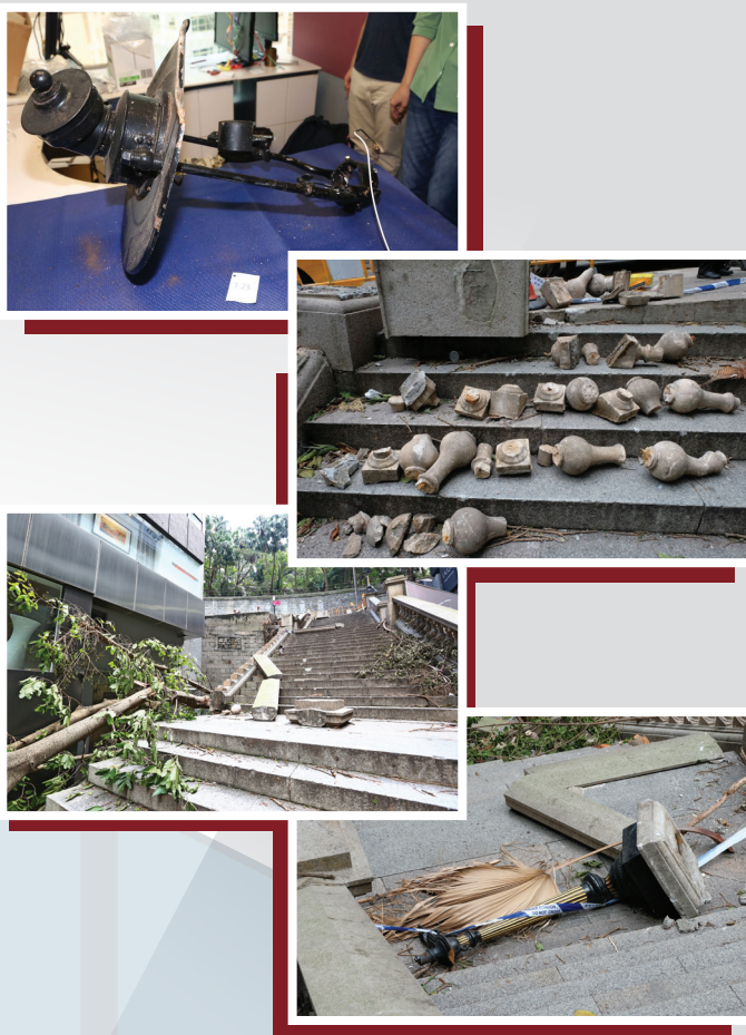
石階、欄杆及煤氣路燈受到嚴重破壞，共檢拾到280件碎片。 The steps, balustrades, and gas lamps were seriously damaged. A total of 280 fragments were salvaged.
