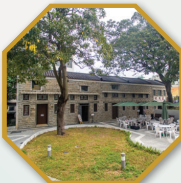
石屋家園 (石屋) Stone Houses Family Garden (Stone Houses)
