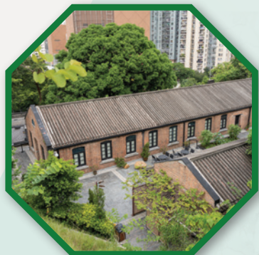
饒宗頤文化館 (前荔枝角醫院) Jao Tsung-I Academy (Former Lai Chi Kok Hospital)
