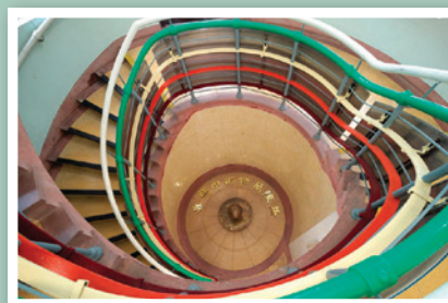
主樓的中央旋轉樓梯及意大利批盪飾面 The central spiral staircase with terrazzo finishes of the main building
