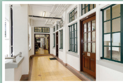
主樓的木門、帶花紋玻璃或普通玻璃的鋼框窗戶及舊式小五金，均保持完好 The timber doors, steel-framed windows with patterned or plain glass panes, and the old-styled ironmongery of the main building are all well maintained
