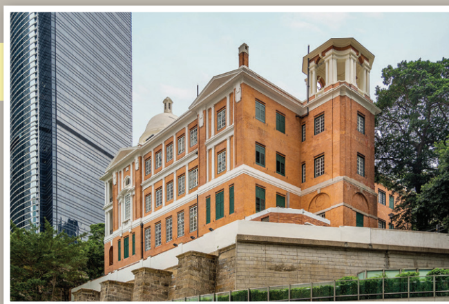
前法國外方傳道會大樓 Former French Mission Building
