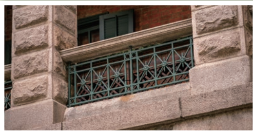
正立面的外廊（上）和扶手裝飾（下）是大樓的建築特色之一。 The verandah (top) and ornamental balusters (bottom) of the front façade are one of the architectural features of the building.
