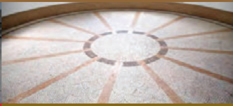
修復後 After restoration
