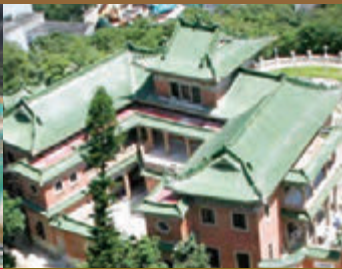
修復後 After restoration
