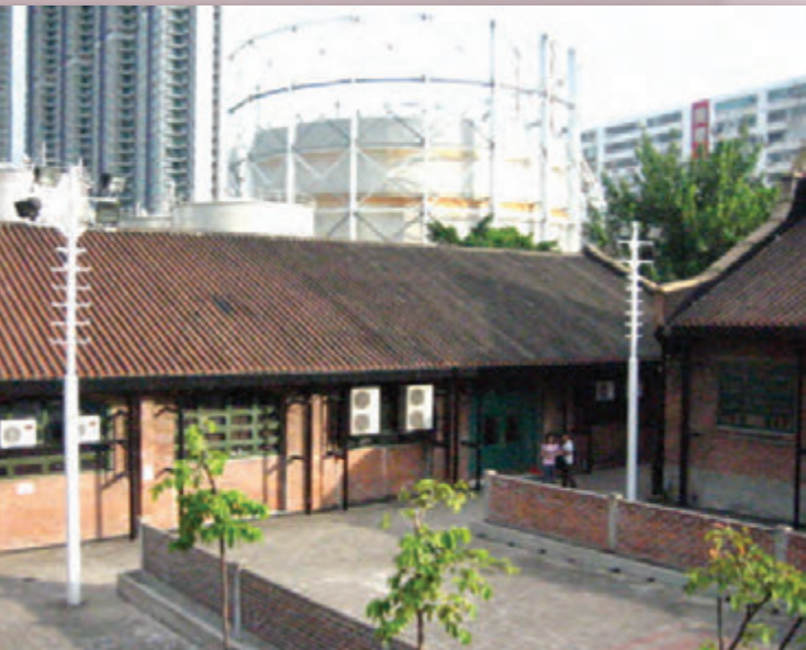
中式瓦片尖形屋頂。 Pitched roof with Chinese-tile.
