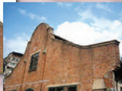
踏步式山牆。 Gable walls with corbelled ends.
