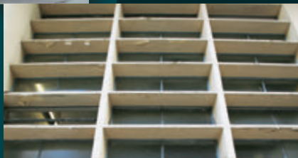
街市的大型玻璃窗及橫向流線型窗戶。 The market building's translucent glass blocks and horizontal streamlined bands of windows.
