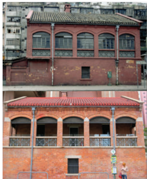
改建前的紅磚屋 (2000年) (相片由古物古蹟辦事處提供) Red Brick Building before conversion, 2000 (photo courtesy of the Antiquities and Monuments Office)
