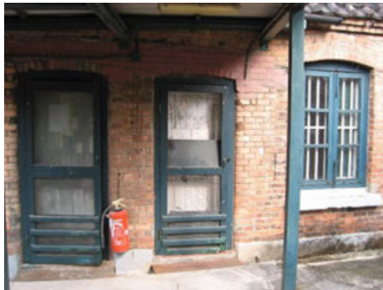
8.4) Wooden doors and granite thresholds to doorways
