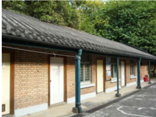
6.2) Chinese tiled pitched roof and verandah with iron posts
