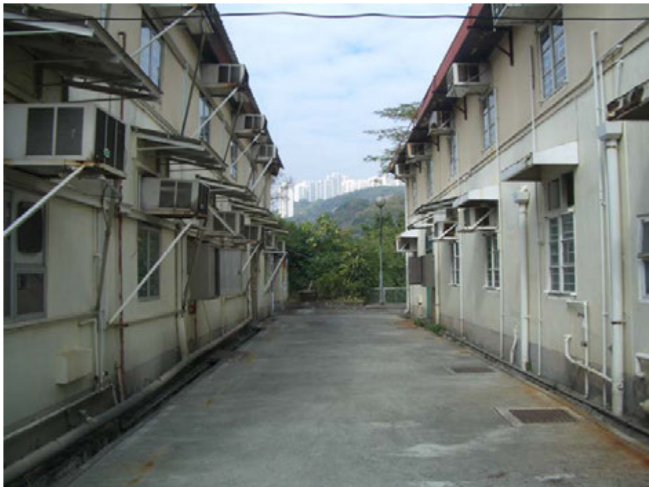
View of blocks at upper section
