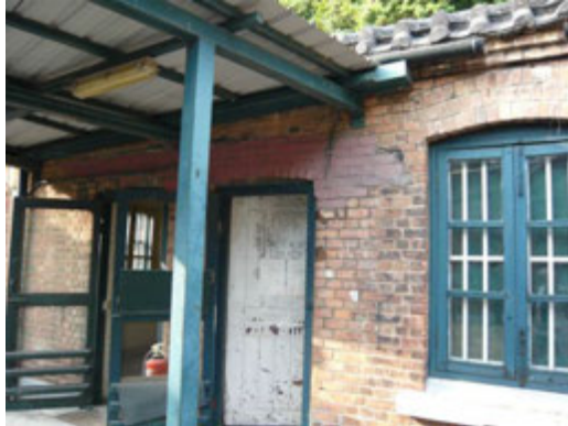
8.3) Wooden casement windows, burglar bars, rendered brick cills and concrete lintels
