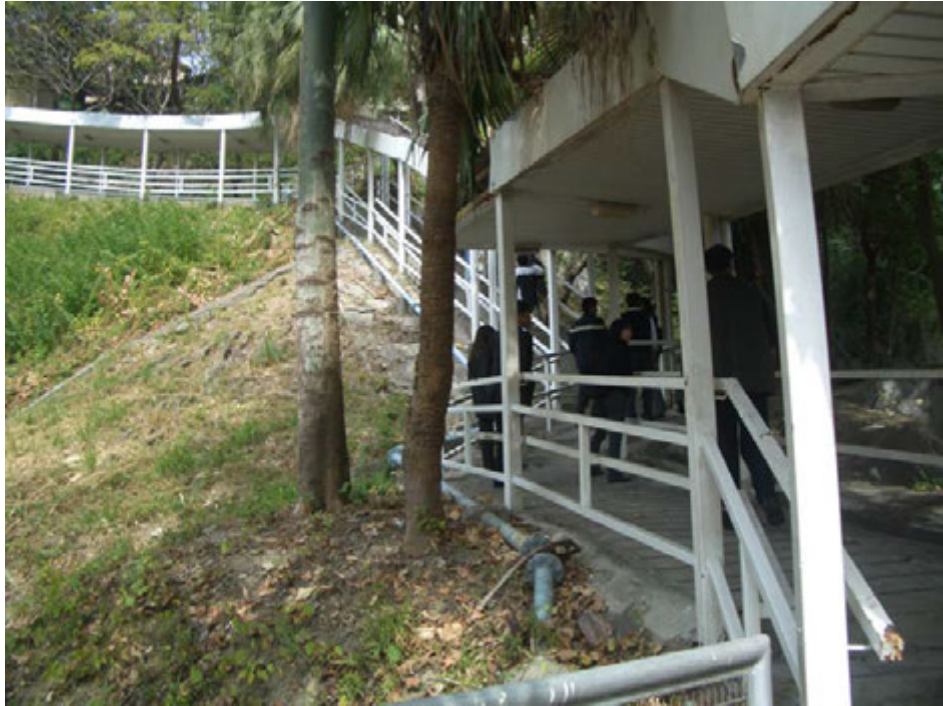
Covered walkway connecting middle section and upper section
