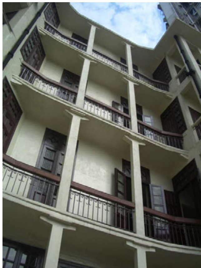
View of west façade of Lui Seng Chun
