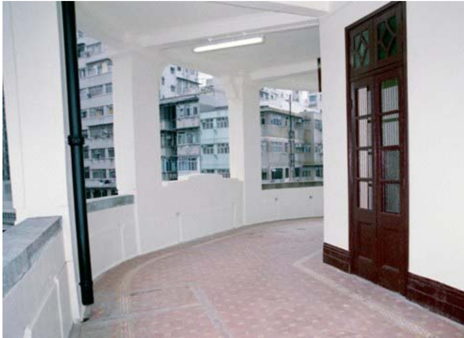
View of verandah
