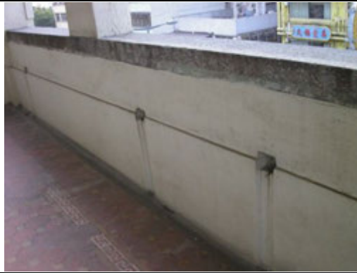
1.7) Drainage outlets at balconies at all floors
