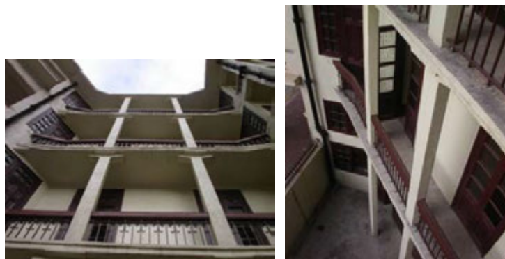
1.9) The Rear verandah with concrete slab and profiled column supports
