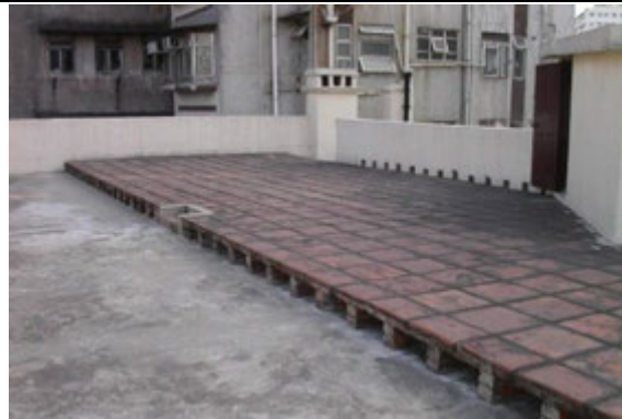
1.10) The main reinforced concrete roof slab together with Canton clay tiled insulating roof on top
