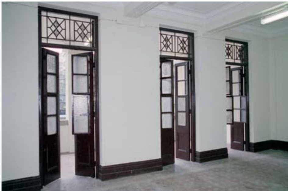
View of timber doors located between room and verandah
