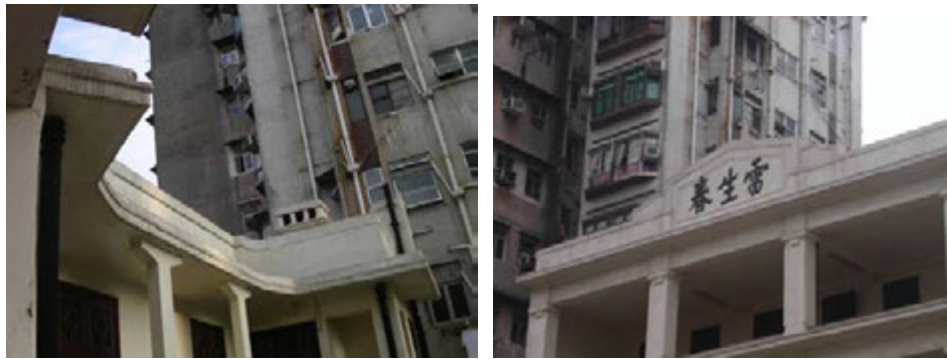
1.8) Canopies projecting from face of parapets at the roof slab level
