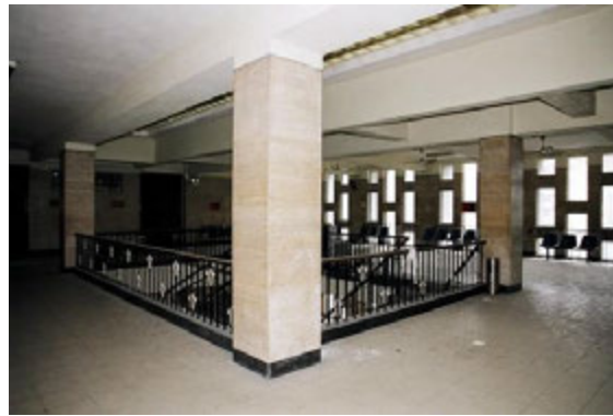
7.3) Marble cladding to walls and columns of Hall
