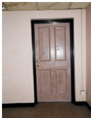
6.7) Original wooden panelled door and frame to staircase off Staff Canteen
