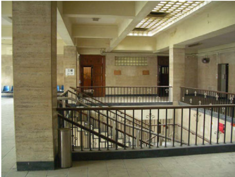
View of balustrade and staircase at 2/F
