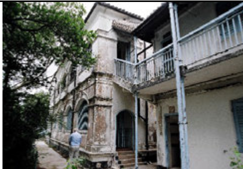
2.7) Connecting bridge and steps to Outhouse
