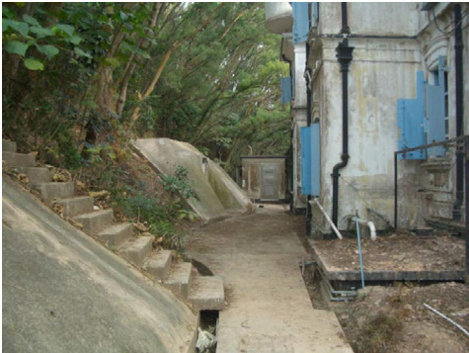
View of footway beside Main Building
