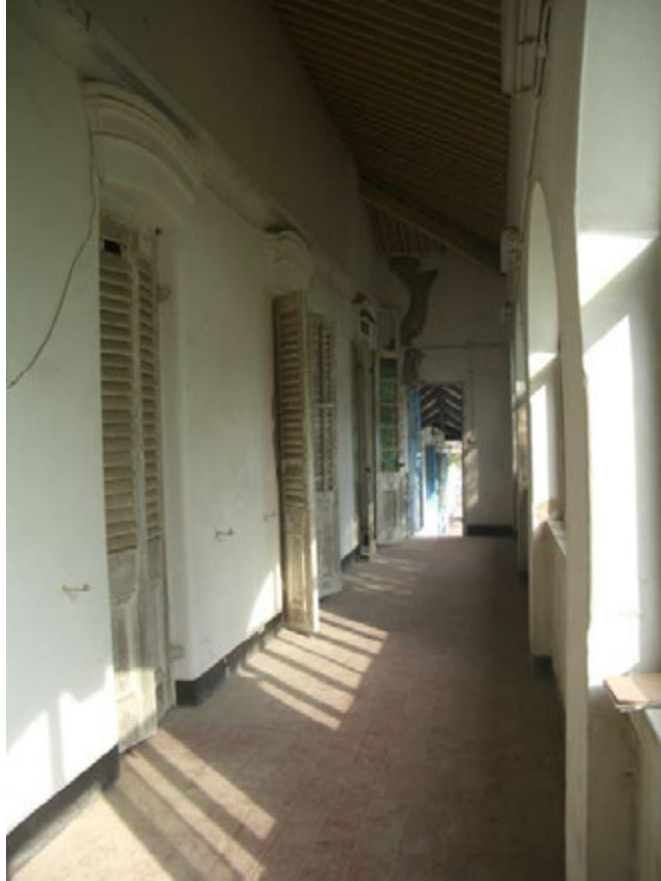
View of verandah at 1/F of Main Building
