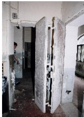
3.9) Steel doors to Charge Room and rear exit on G/F
