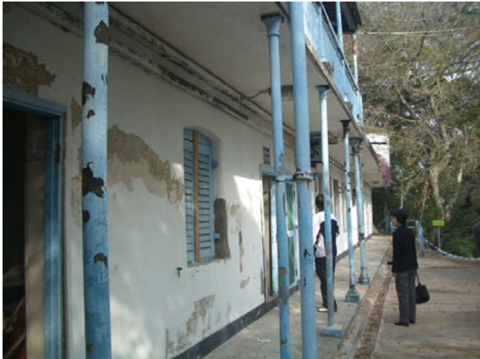
View of verandah at G/F of Outhouse
