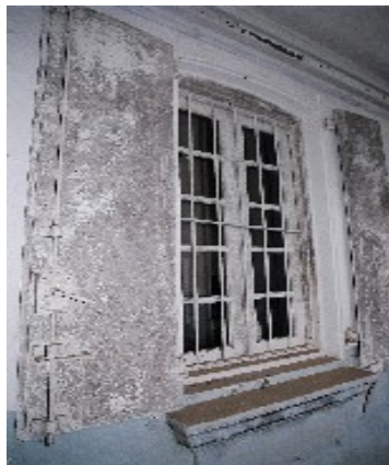
3.2) Original wooden casement windows, burglar bars and steel shutters to windows to rooms on G/F
