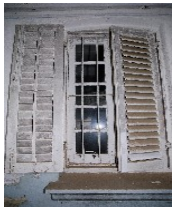
3.2) Original wooden casement windows, burglar bars and steel shutters to windows to rooms on G/F
