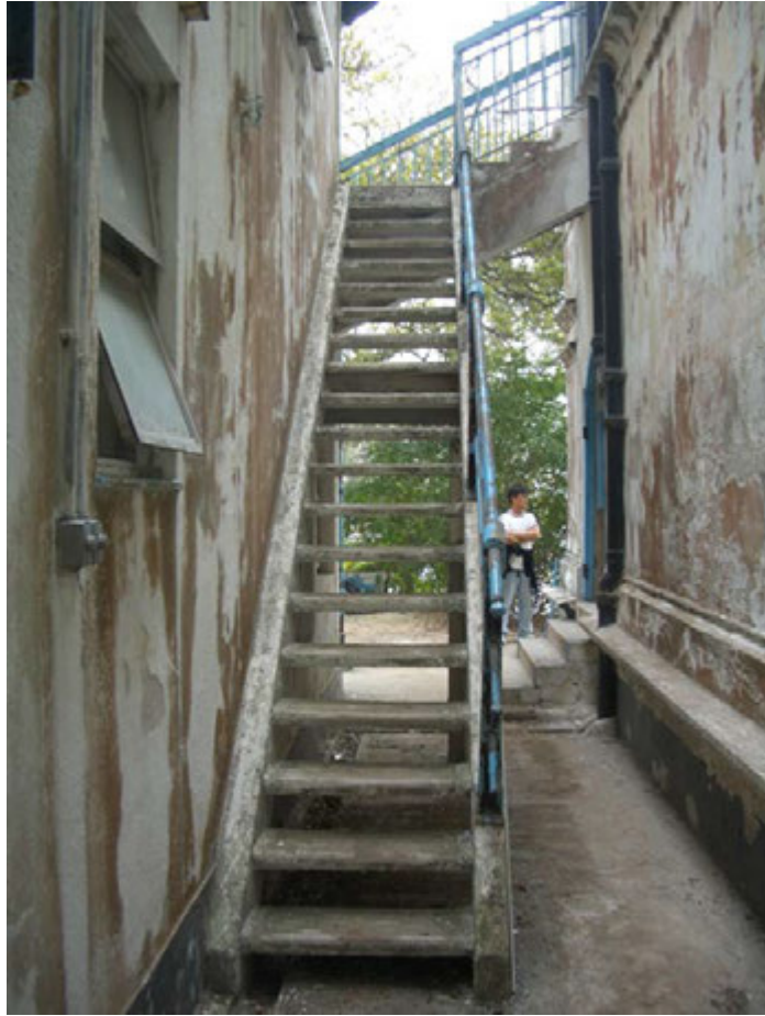
View of external staircase between Main Building and Outhouse
