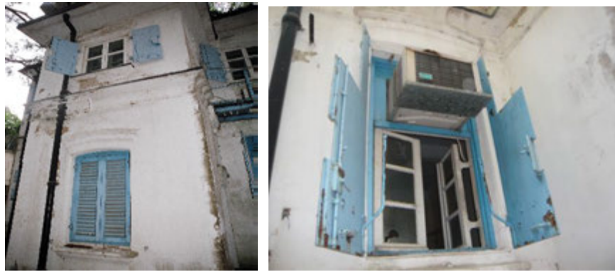
2.5) Original wooden casement windows and jalousies, some with steel shutters
