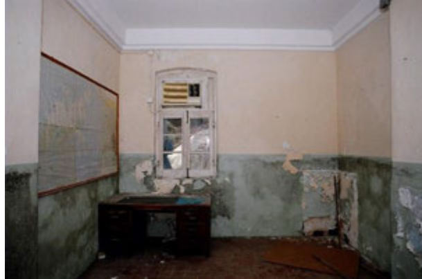
3.1) Plastered and painted walls and ceilings to rooms on G/F
