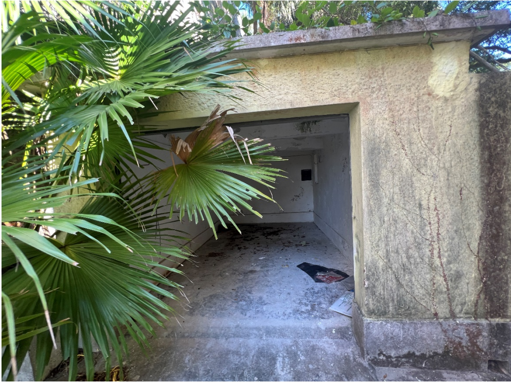
2.7 车库大楼的整体景观
