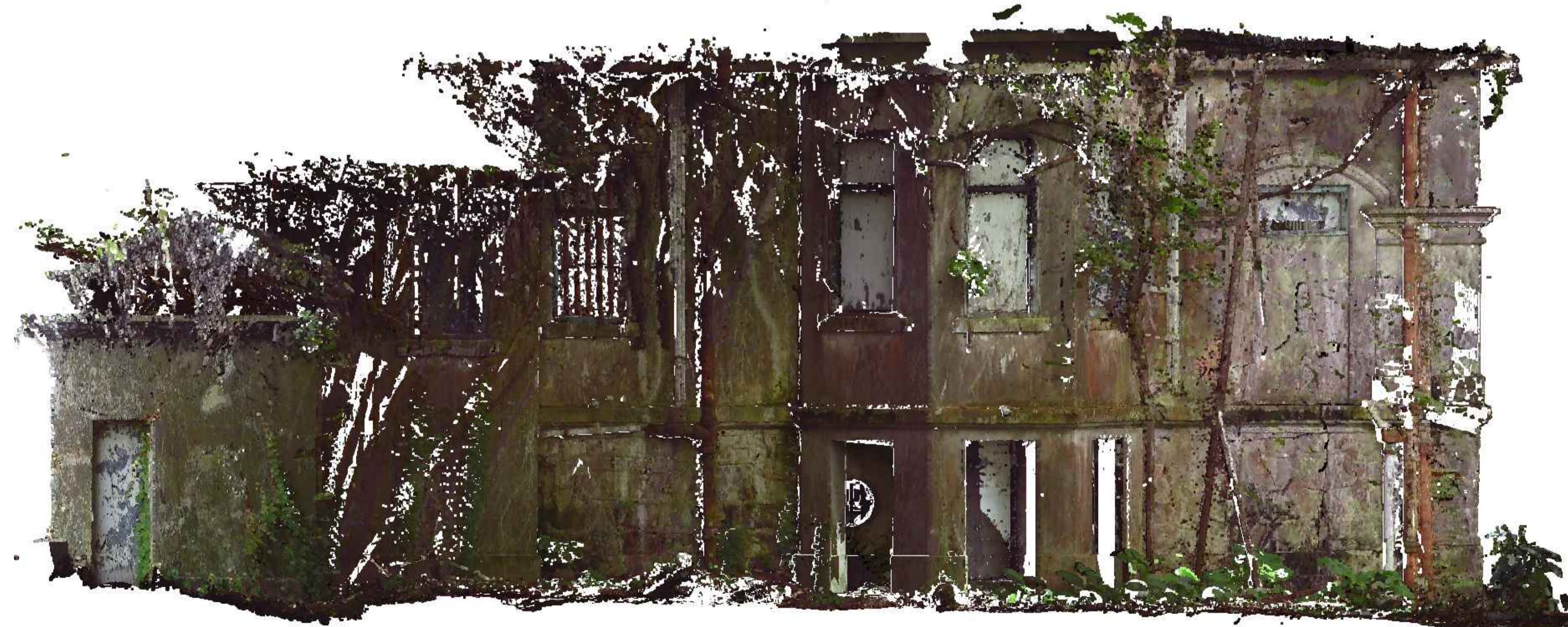
POINT CLOUD OF NORTH ELEVATION
